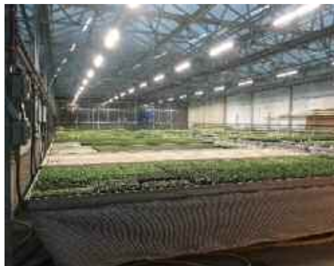
Peace Tree Farms installed the VYPRx Plus System LED lights from Fluence Bioengineering, which they are leasing.
