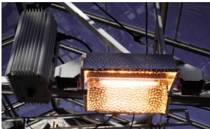
A double-ended high-pressure sodium (HPS) lamp that shows the unique connection of the bulb in the fixture. HPS lights are a good choice for large greenhouses full of plants. The light from 1,000-watt HPS fixtures is so concentrated that the fixtures need to be placed higher, so the light is distributed uniformly over a larger area.
